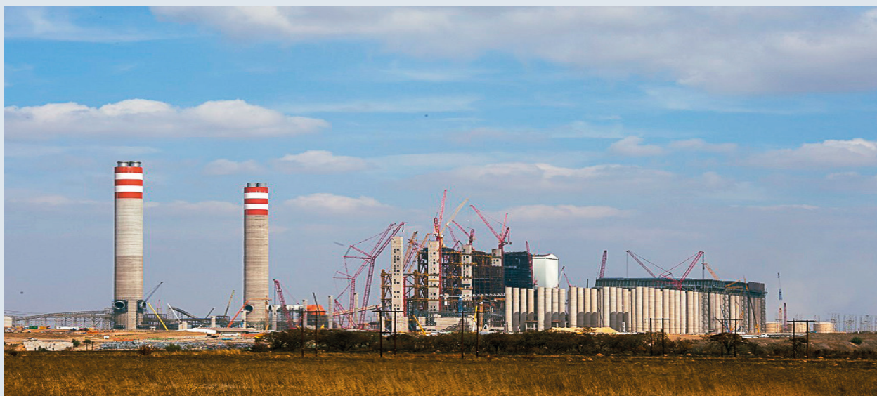
Swiss engineering firm ABB Group was contracted to work at Kusile in 2015.
